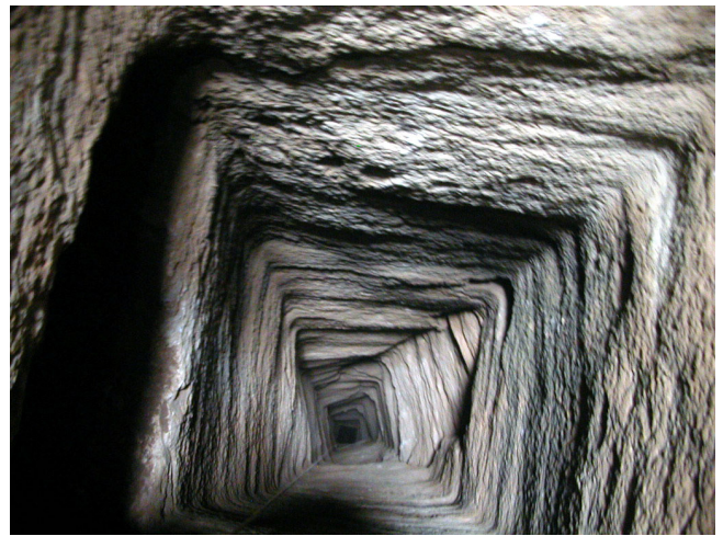
Figure 10. Typical twisted shaft Nic 4, called Persephone, in the Spitharopoussi area. Note that the twist occurs either regularly or in sections from top to bottom.
