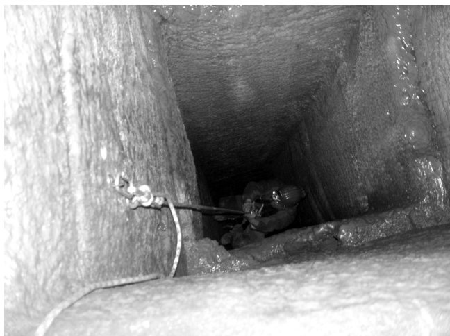
Figure 13: Shaft Spi 2, exploration of the air duct.
