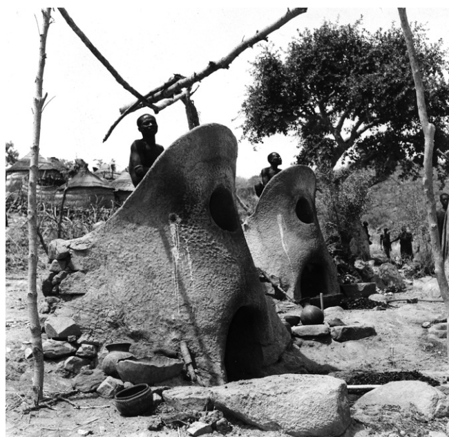
Figure 2 (below): Teleki furnaces, estimated height c2m. According to Gardi the men are singing and pumping the bellows, but it is far from clear that a smelt is in progress (Gardi 1953, Plate 54). Photo René Gardi 1953/77/12 by kind permission of Bernhard Gardi.
