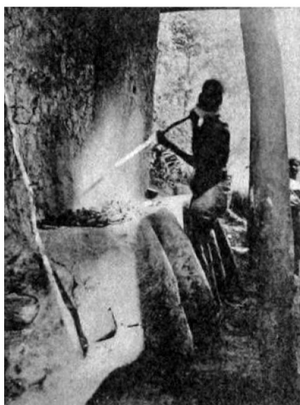
Figure 3: Iron smelting demonstration at Hatarabage held for Ananda Coomaraswamy. A: the workshop with two furnaces and the bellows operator visible behind the wattle and daub wall separating the bellows from the furnace. B: detail of the smelter, possibly with his foot on a stepping stone at base of structure. The two large shoulder stones appear to be plastered into the structure.
