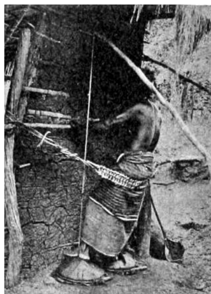
Figure 4: A: the foot bellows used in the Coomaraswamy smelting demonstration, showing their construction. B: the operation of similar bellows at Mawalgaha where Coomaraswamy recorded a demonstration of crucible steel making.
