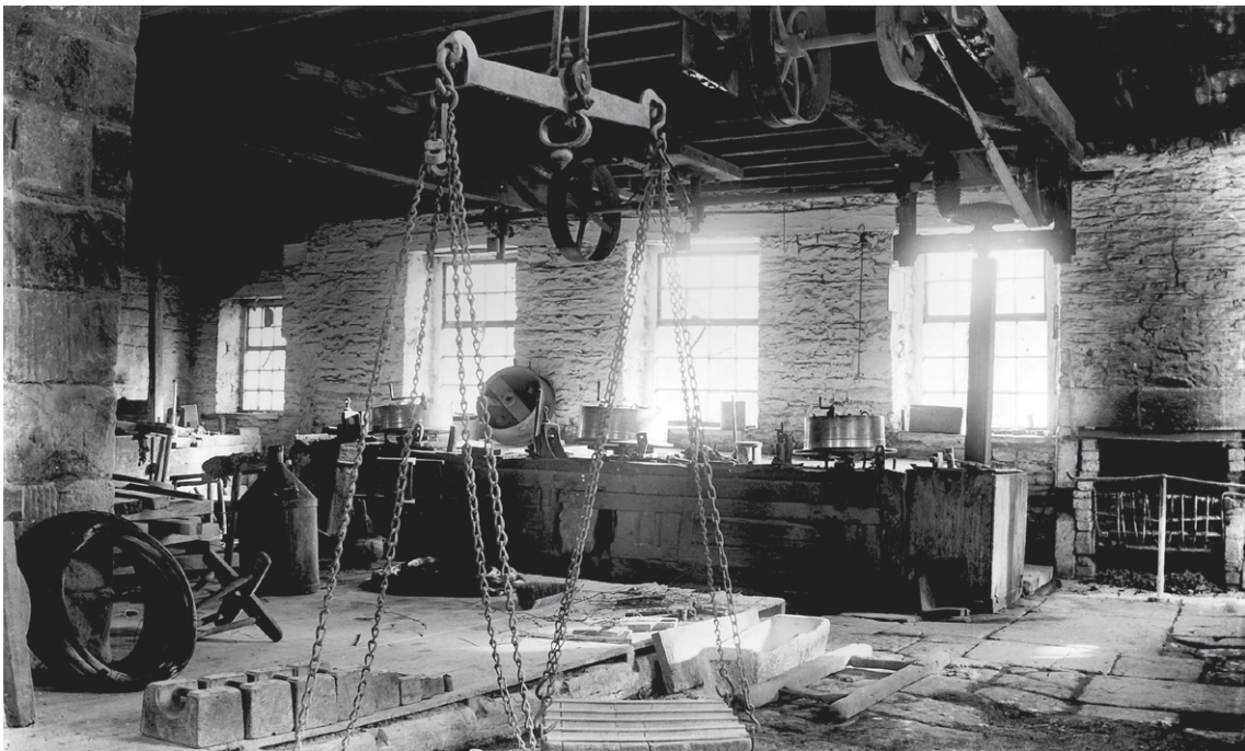
Figure 5: The wire-drawing bench in Fig 4, from a different position at a different time, showing weighing scales and weights in the foreground, a barrel of soft soap near the left-hand end of the bench, and coils of wire.
