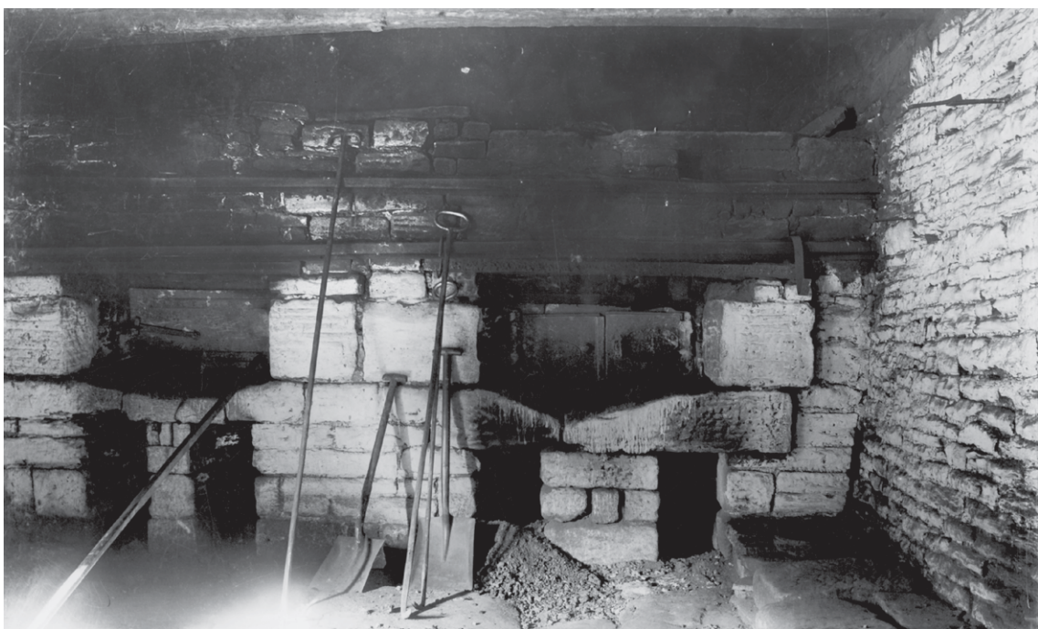
Figure 7: Annealing furnaces. The closed doors can just be made out in the lower part of the shadows.
