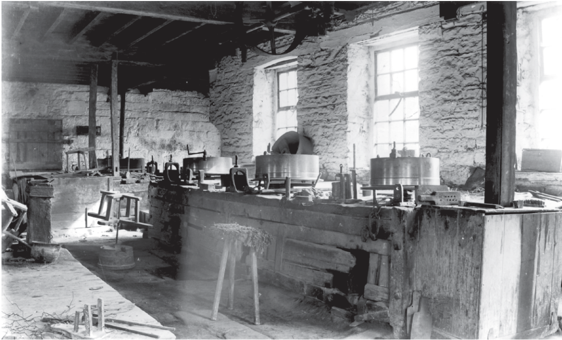
Figure 4: This interior view shows most of the equipment required for drawing steel wire by water power. The wire-drawing bench has three blocks (drums) with wire in position. An empty swift is on the floor near the far end of the bench. A wortle plate, of typical shape with drawn neck, rests on edge on the nearest end of the bench, and the ends of two more are just visible on the floor, partly out of the photograph, in the foreground. Another wortle plate is set up on the bench beyond the nearest drum. Clamps, in which wortle plates could be fixed, are fitted along the edge of the bench. The drive shaft from the water wheel is concealed within the bench, but an encased vertical drive shaft to benches on the floor above can be seen at the right hand of the image, near the end of the bench. Below this casing, close to the floor, and to the left of the two wortle plates, a clutch pedal is just visible, controlling the drive to the blocks.
