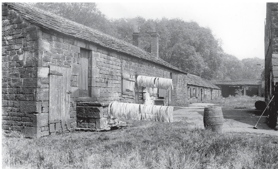
Figure 9: Reels of wire, coated with lime after annealing, drying outside the mill.
