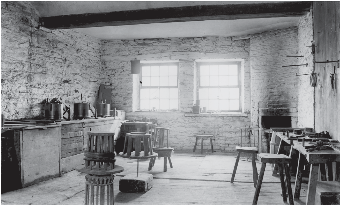
Figure 11: This is thought to be the first-floor wire-drawing shop at Thurgoland Old Mill. Blocks can be seen on the bench to the left, filled with wire, and empty swifts are prominent. The small bench on the right is probably for the hand-drawing of fine wire.
