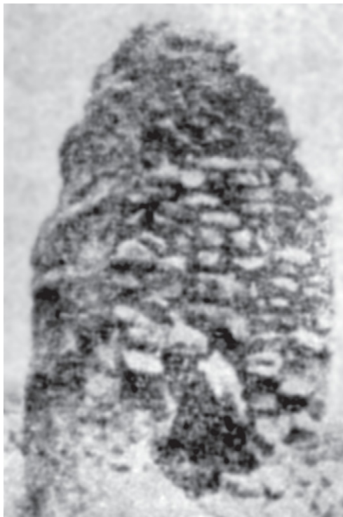
Figure 2: A Song-period blast furnace, still standing at Kuangshancun near Handan, Hebei. Left: Photograph, originally in Guangming ribao , 13 December 1959, here reproduced from Liu Yuncai 1978, 23, fig 8. Right: Liu Yuncai's reconstruction of the furnace. Cf Figures 3–4.
