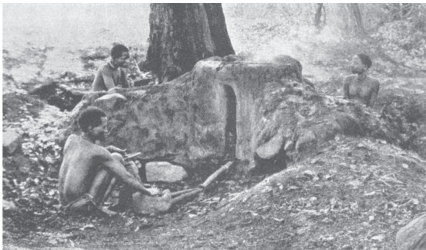
Figure 2: A photograph taken by M H Gros of an iron smelting furnace on the farm Schuynshoogte, bordering Schiel on the western side (from Junod 1927, 139). Note the bag bellows, the antelope horns connecting them to clay tuyères, the round furnace with three characteristic vertical slits, and the squatting position of the bellows blowers.
