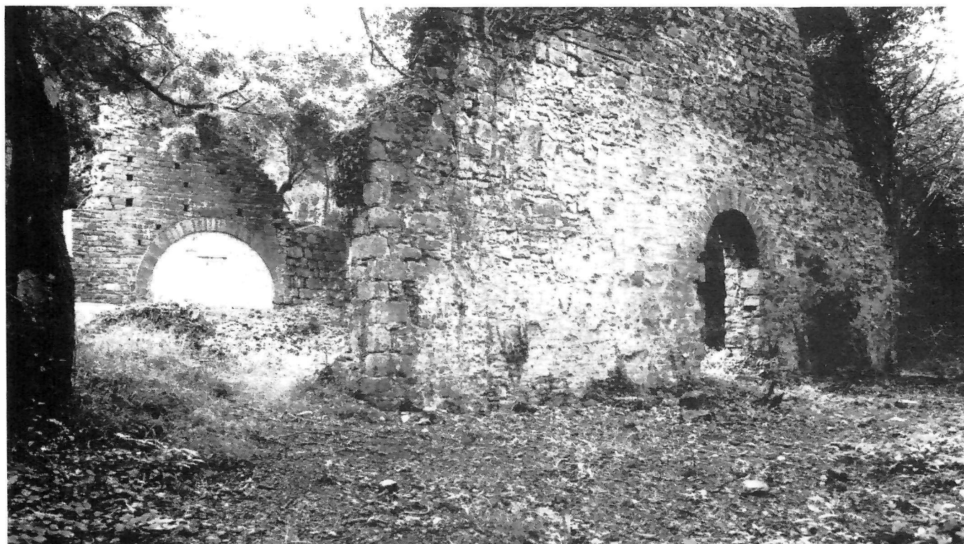
Figure 2. Bedford's Ironworks at Cefn Cribwr from the entrance. The furnace is on the left and the gable end of the cast house on the right. (Photo P. Hutchison).
