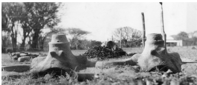
Figure 5: Two Njanja iron-smelting furnaces constructed at Charter Range for the visit of His Royal Highness, the Prince of Wales, in the early 1920s. Note the general similarity in both size and shape to the furnace shown as a scaled drawing in Figure 4, the side accessories, plus cicatricization marks below the breasts, and the front rake hole beneath a low arch, with a charcoal (?) stockpile at the rear. The air blast, provided by two men operating four goatskin bellows, would have been directed through two horizontal tuyeres inserted into moulded holes at the rear of each furnace. (Photo: National Museums and Monuments of Zimbabwe).
